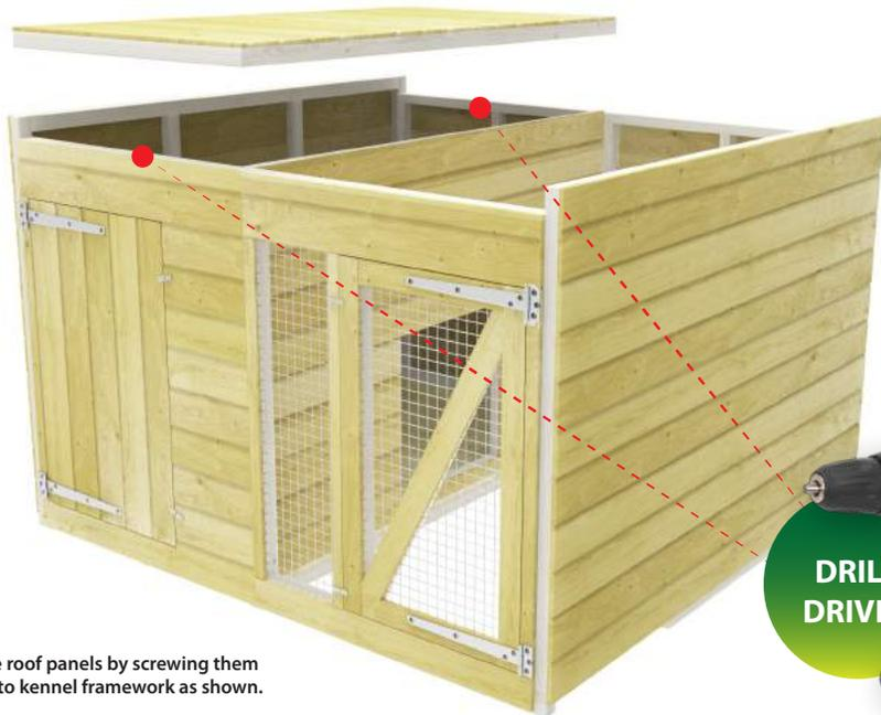
Secure roof panels by screwing them down to kennel framework as shown.
