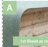
**17a.** Apply the roof felt as shown. Apply lower levels first to create correct rain run off positions.
