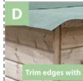
**17c.** Trim down excess felt with a stanley knife. Remember to overlay the 1st felt to avoid rain leaks.
