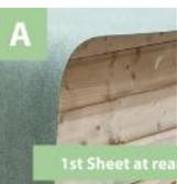
**16a.** Apply the roof felt as shown. Apply lower levels first to create correct rain run off positions.
