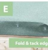
**16d.** Tuck and fold edges neatly and tack in place to hide any loose edges. Check that all areas are covered and there are no holes to avoid any rain water getting through your felt roof.
