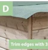
**16c.** Trim down excess felt with a stanley knife. Remember to overlay the 1st felt to avoid rain leaks.
